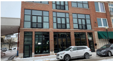
BUREAU GRAVITY FAÇADE CONDITION ASSESSMENT + REHABILITATION AURORA, ILLINOIS COMMERCIAL SECTOR / COMPLETED 2015
