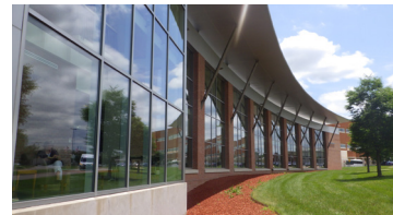
US DEPARTMENT OF VETERANS AFFAIRS ASCE 41 SEISMIC EVALUATION MULTIPLE SITES THROUGHOUT THE MIDWEST HEALTHCARE SECTOR / COMPLETED 2018
