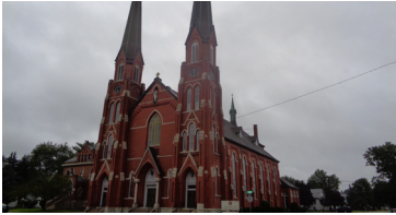
PEORIA CATHOLIC DIOCESE ST. HYACINTH CHURCH STEEPLE AND STRUCTURE ASSESSMENT + REPAIR COSTS LASALLE, ILLINOIS RELIGIOUS SECTOR / COMPLETED 2019
