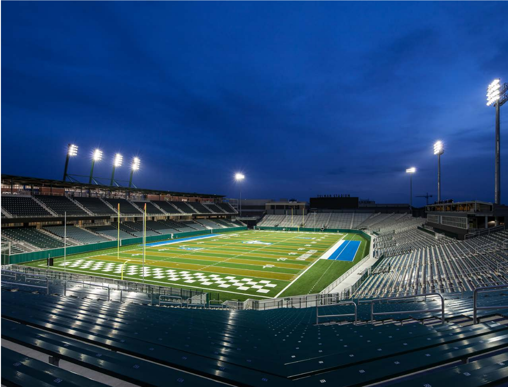
TULANE UNIVERSITY YULMAN STADIUM STRUCTURAL ENGINEERING
