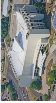
INDIANA UNIVERSITY ASSEMBLY HALL REROOF BLOOMINGTON, INDIANA CONSTRUCTION COST $2.71 million YEAR COMPLETED 2011
