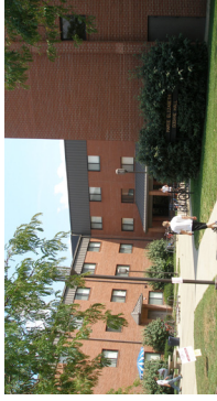
VINCENNES UNIVERSITY MULTIPLE ROOF CONDITION ASSESSMENTS VINCENNES, INDIANA CONSTRUCTION COST N/A YEAR COMPLETED 2007
