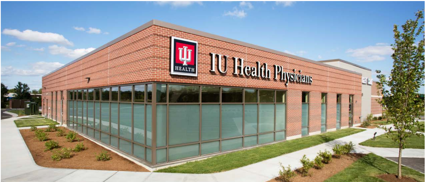
IU HEALTH NOBLE WEST MEDICAL OFFICE BUILDING NOBLESVILLE, INDIANA
